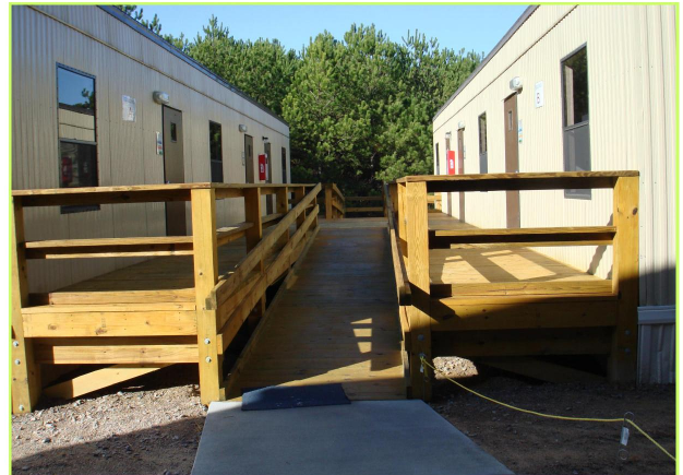
Modular Classroom and Handicap Access Installation
